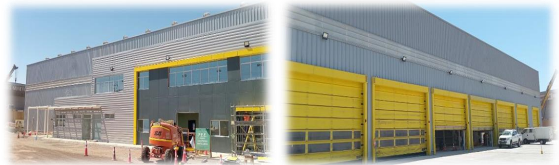
Finning's Newly Built La Negra Service Shop
