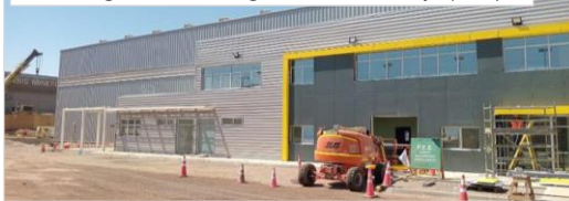
In Progress, La Negra Service Shop (1/2)
