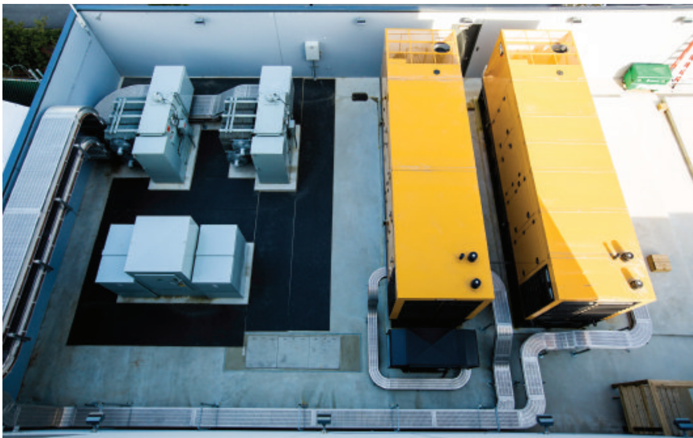
With space at a premium, Global Relay and Finning Canada worked together to make sure the generator sets and UPS systems would fit in the available footprint. The site has two gen-sets installed with two more on the way. A fifth can be installed if demand warrants.
