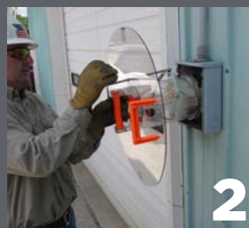
2 Closing non-conductive jaws with actuating rod
