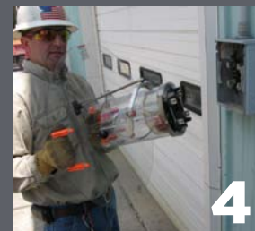
4 Meter removed from socket base
