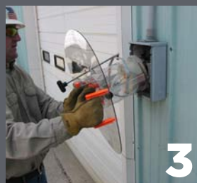
3 Removing/pulling meter
