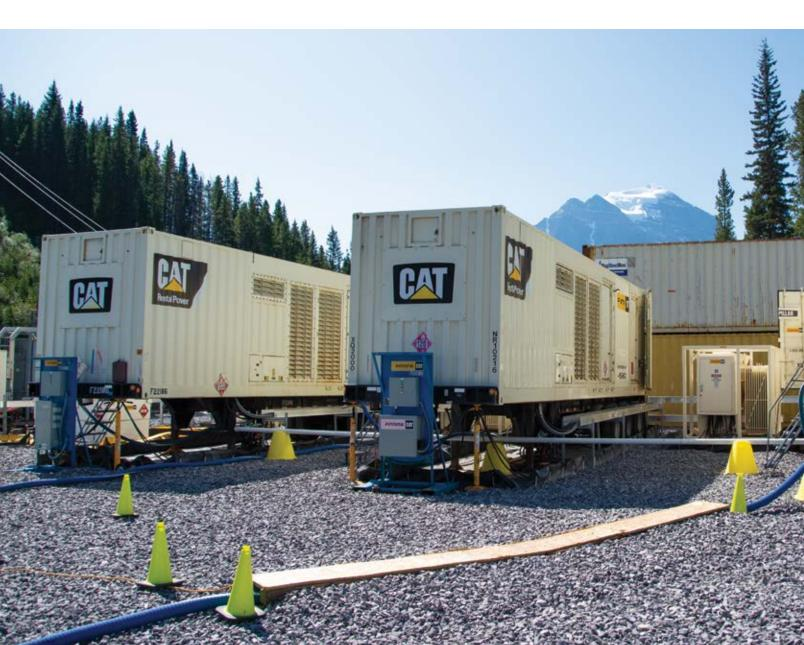
sets, which ran 24/7 and were connected to an AltaLink substation.
