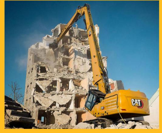
The 50-tonne class ultra-high reach demolition excavator comes with two UHD front options, providing a maximum stick pin height of up to 25m (82 ft), and features a Falling Objects Guard Structure (FOGS), including front and roof laminated glass with a P5A impact rating. The UHD cab tilts up to 30 degrees for excellent visibility to the stick nose to give the operator a more productive and comfortable working position.
