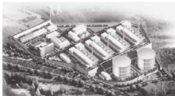
Figure 10: Jingcheng CMM 120 MW Power Project
