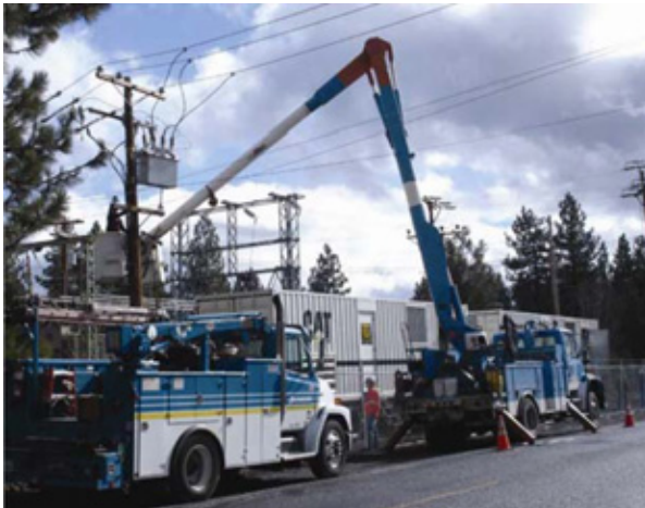
Figure 1: Cat® XQ2000 Power Modules in Chester
