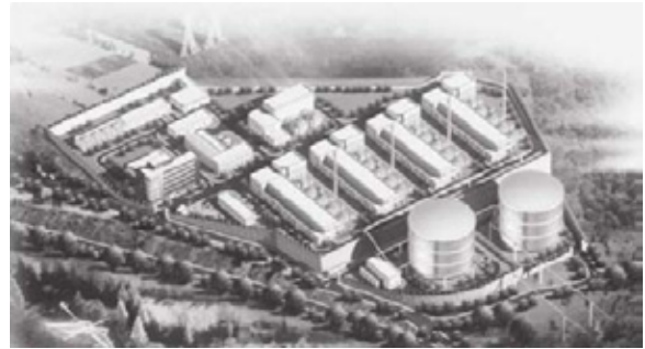
Figure 10: Jingcheng CMM 120 MW Power Project
