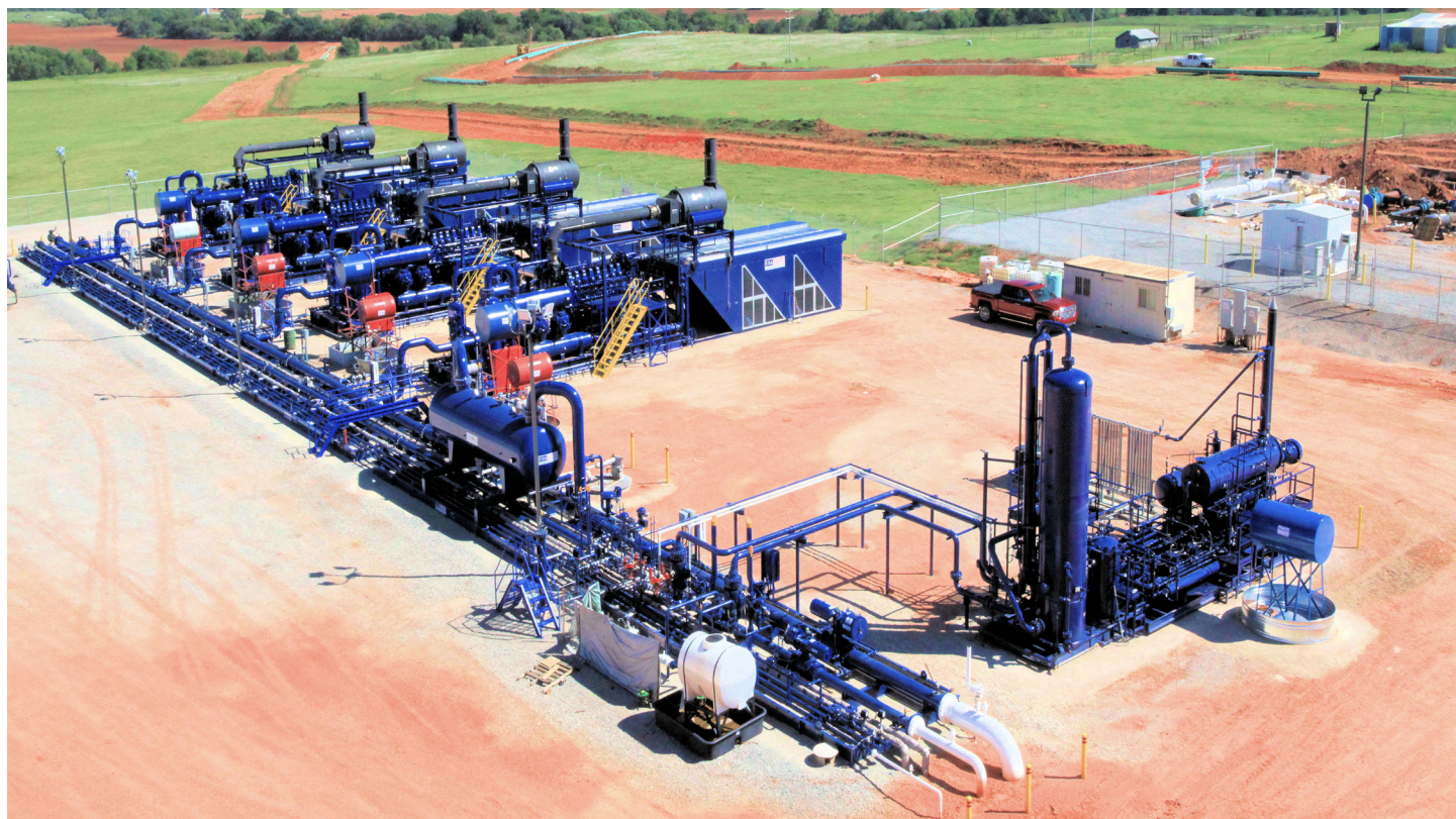
Compressor Station - USA Compression Partners, LP Powered by G3608 A4 engines
